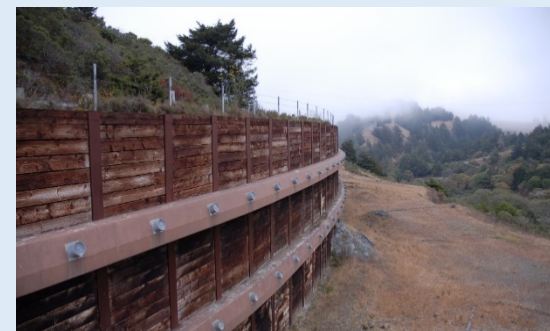
Soldier Pile Retaining Wall on HWY 1
